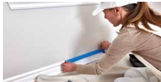
Protection with painter's tape
